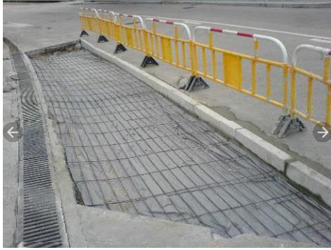
(5) Concrete paving
